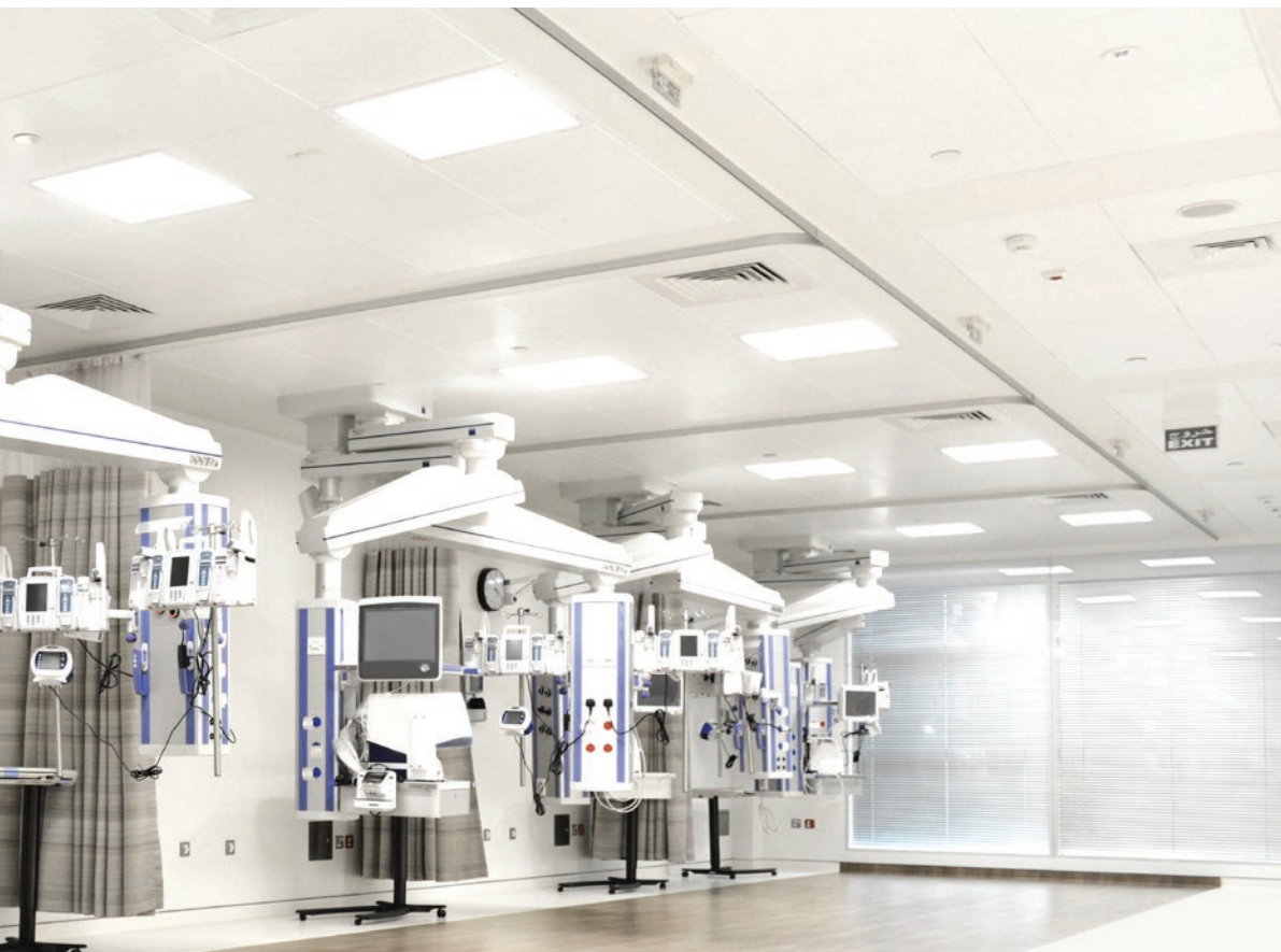
Hamad General Hospital, Doha (Qatar)
