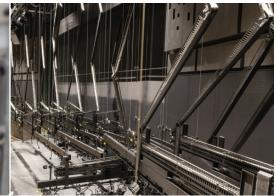
Our Cable Management solutions combine decades of knowledge in UL-Listed circuit and data wireways with the modern needs of compact and safe-running cable technologies. Hoists with Cable Management can raise and lower fixtures for focusing and maintenance without unsightly spools of cables suspended in the air, and without sacrificing space.
