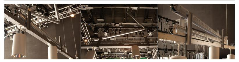
ETC's Houselight Pantograph offers a sleek solution for dressing power and data cables to your flown distribution. It is a unique trough that can support 50lbs between lift lines without a pipe batten for direct attachment of houselight fixtures.
